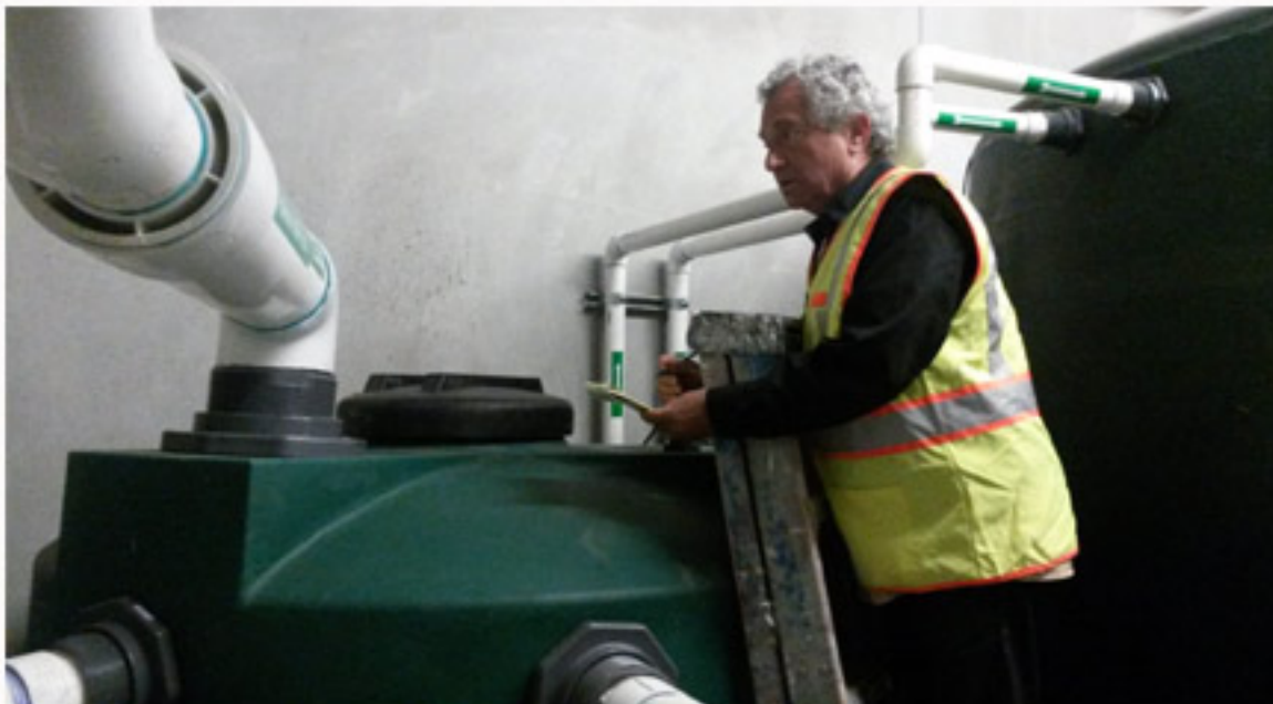
Bobby inspecting the tanks after their installation
